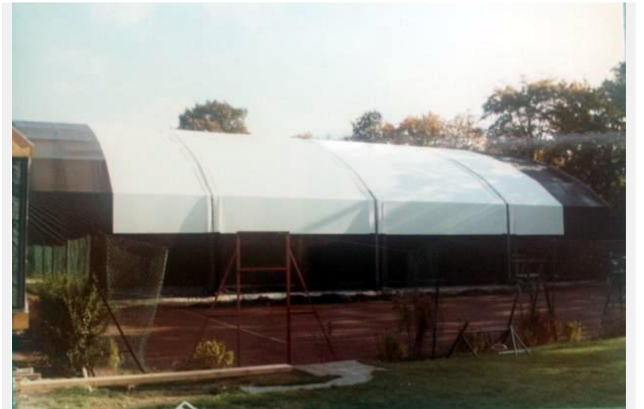
Construction of the new sports hall
