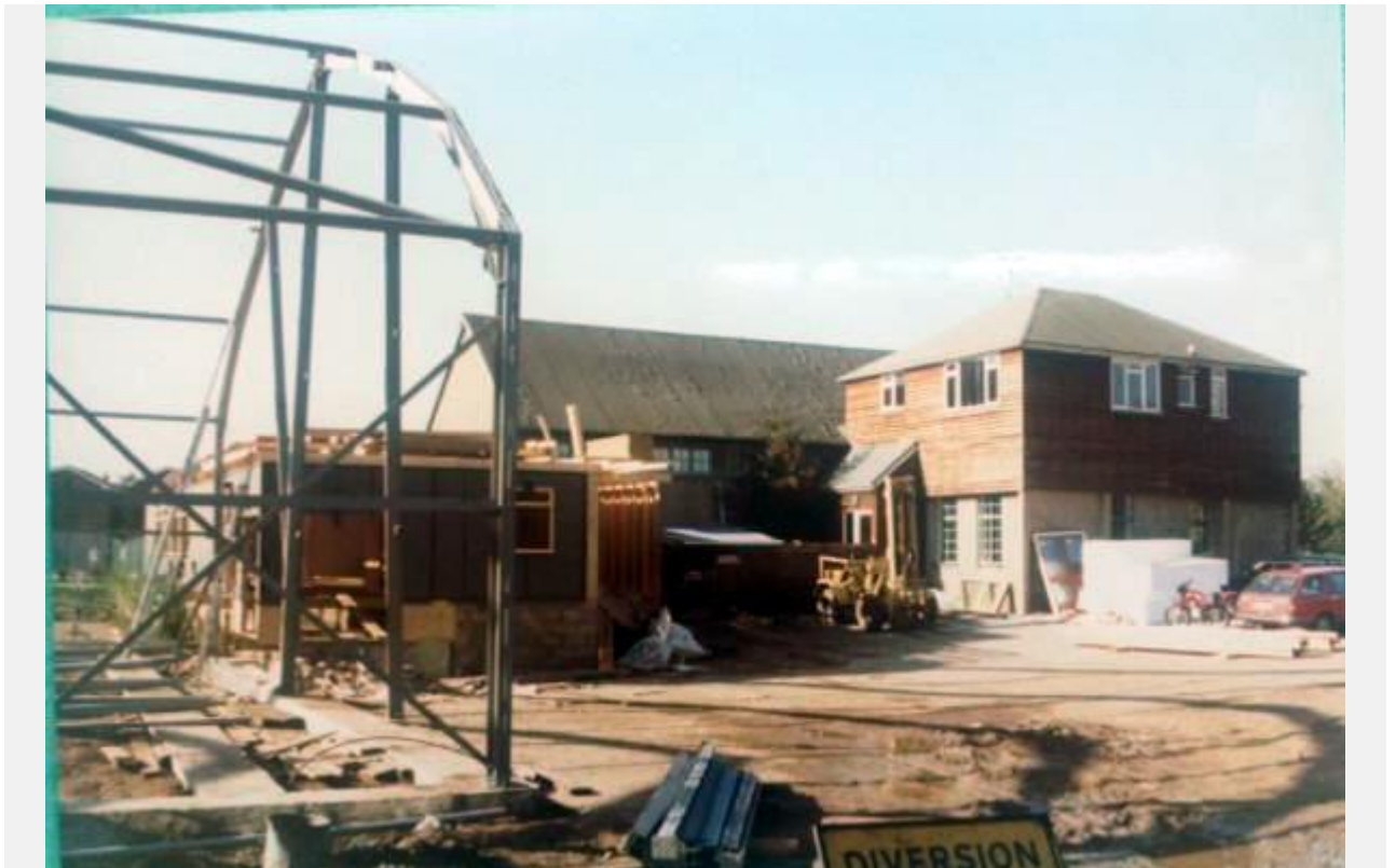
Construction of sports hall and new lounge, office and entrance
