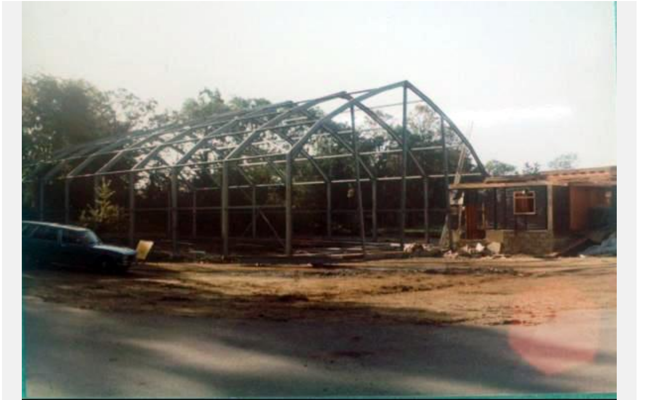
Construction of the new sports hall
