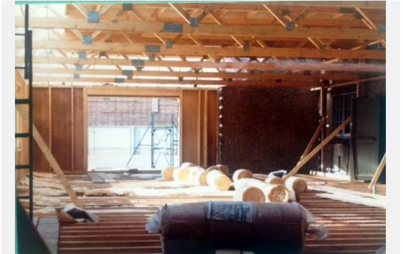
Insulation going into the floor of the new lounge
